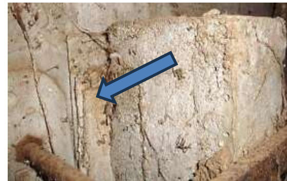
Above: Cement sheet packing (left) in concrete foundations.
