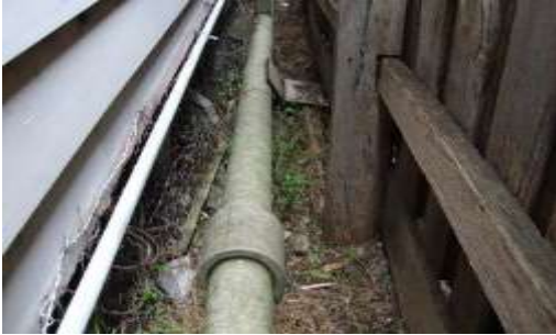
Above: Asbestos cement mains drain pipe.
