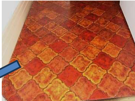
Above: Example of asbestos backed vinyl flooring. Right: White asbestos paper backing.
