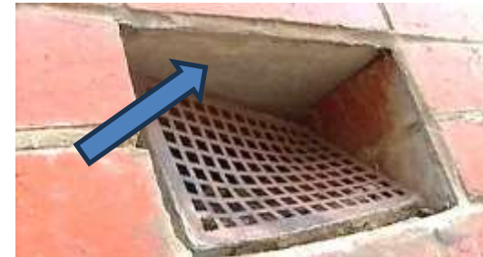
Right: Cement sheet shuttering to top of wall vent.
