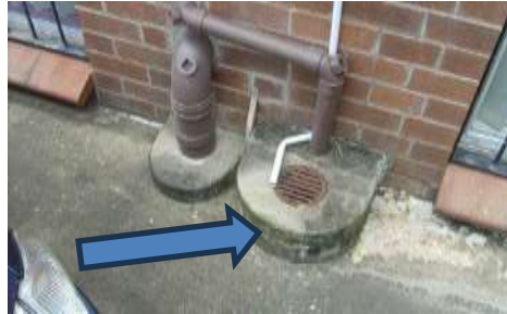
Right: Asbestos cement drain collar (filled with non-ACM).
