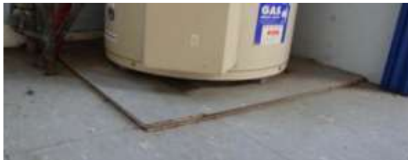
Above: Example of asbestos backed vinyl flooring. Right: White asbestos paper backing.
